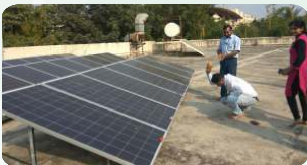
Installation of 8KW Grid Tided Solar Power Plant
